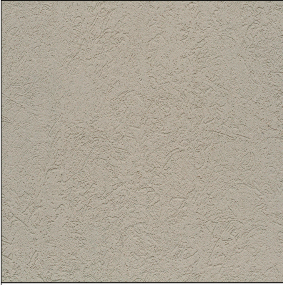
SOFFITS: PLASTER CEMENT W/ EARTH TONED FINISH, EXACT SHADE TBD.
