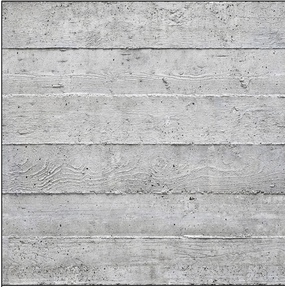
RETAINING WALLS: BOARD FORMED CONCRETE
