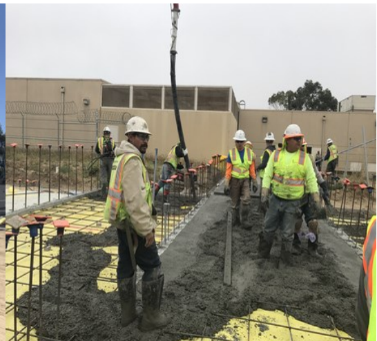
Corridor Concrete Placement
