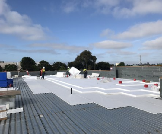
Building A Roofing Insulation
