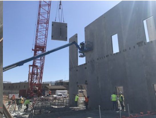
Precast Wall Panel Placement
