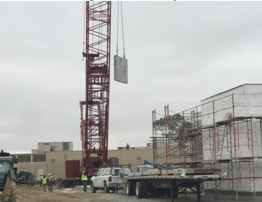
First Panel Lift
