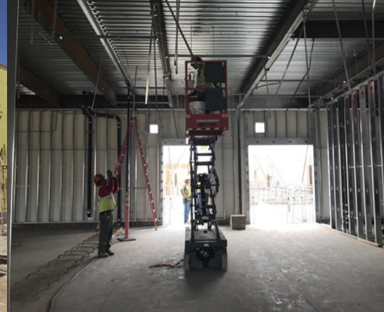
Building A Installing Hangers for MEP
