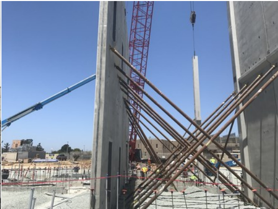
Wall Panel Bracing
