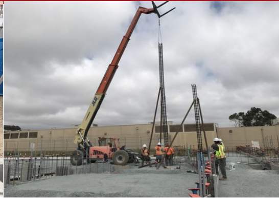
Cast In Place Concrete Columns
