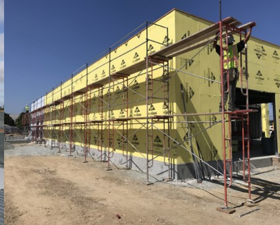
Building A Scaffolding
