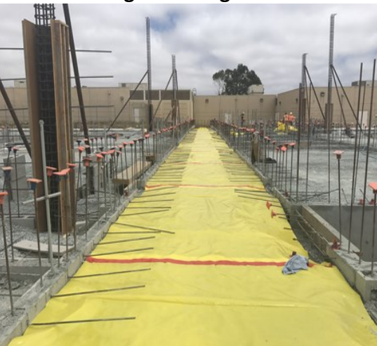
Connecting Corridor Vapor Barrier
