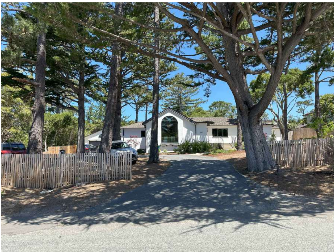
STREET VIEW OF (E) HOUSE & GARAGE
