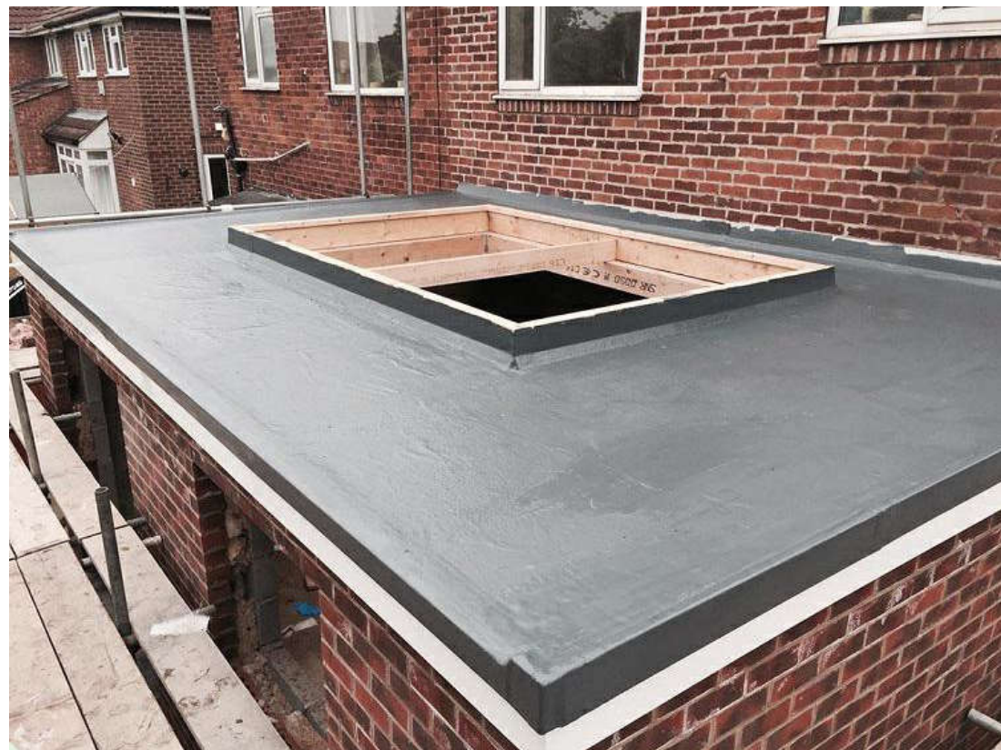
RUBBER MEMBRANE ROOF
