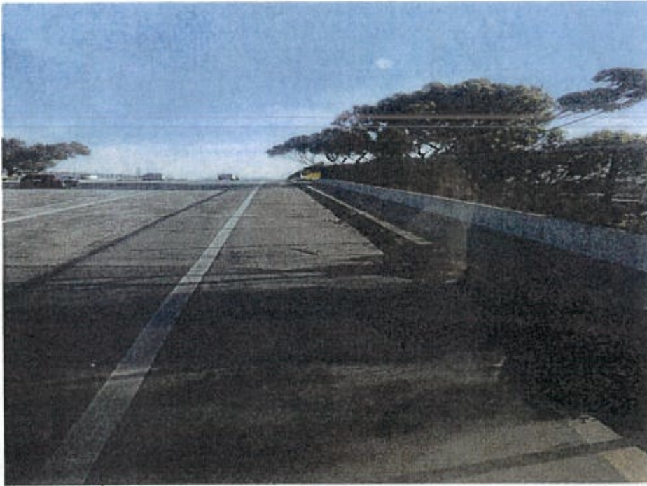
BEFORE: Davis Rd. Bridge 5-1-2020 (SAMPLE)
