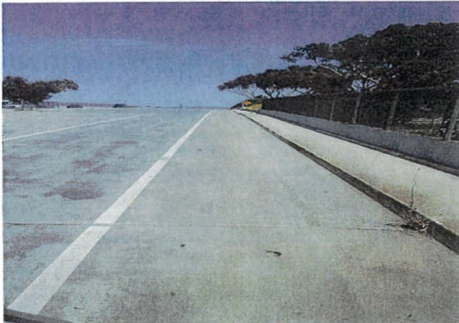
AFTER: Davis Rd. Bridge 5-1-2020 (SAMPLE)
