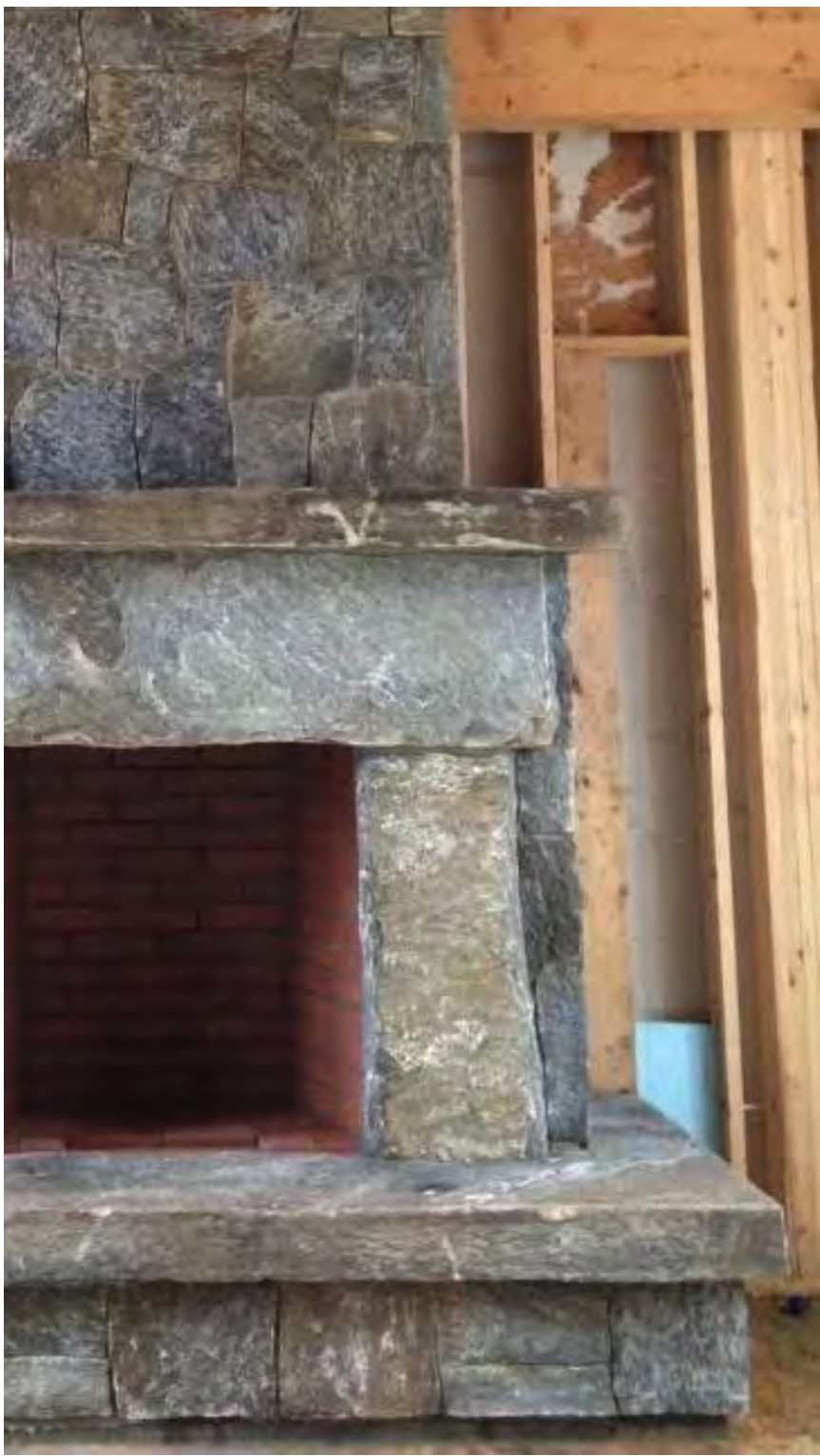
STONE: CHAMPLAIN STONE - 1763 GRANITE, 3"-5" THICK VENEER IN "LEDGESTONE" LAY
