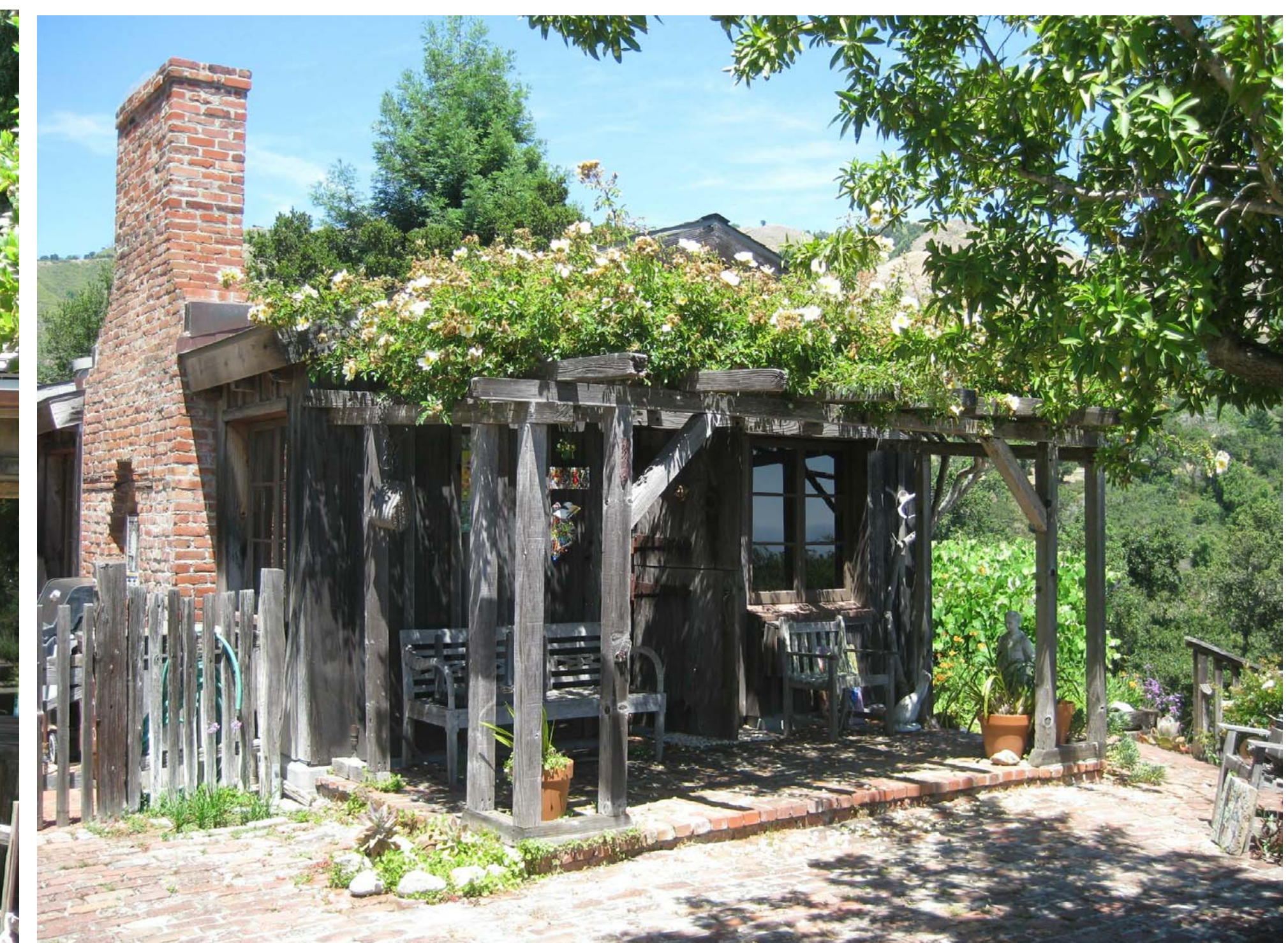
MAIN RESIDENCE - WEST ELEVATION
