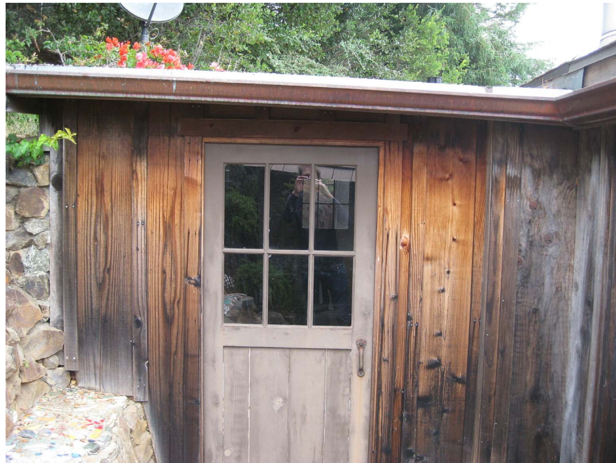
MAIN RESIDENCE - BACK PORCH - N/W ELEVATION
