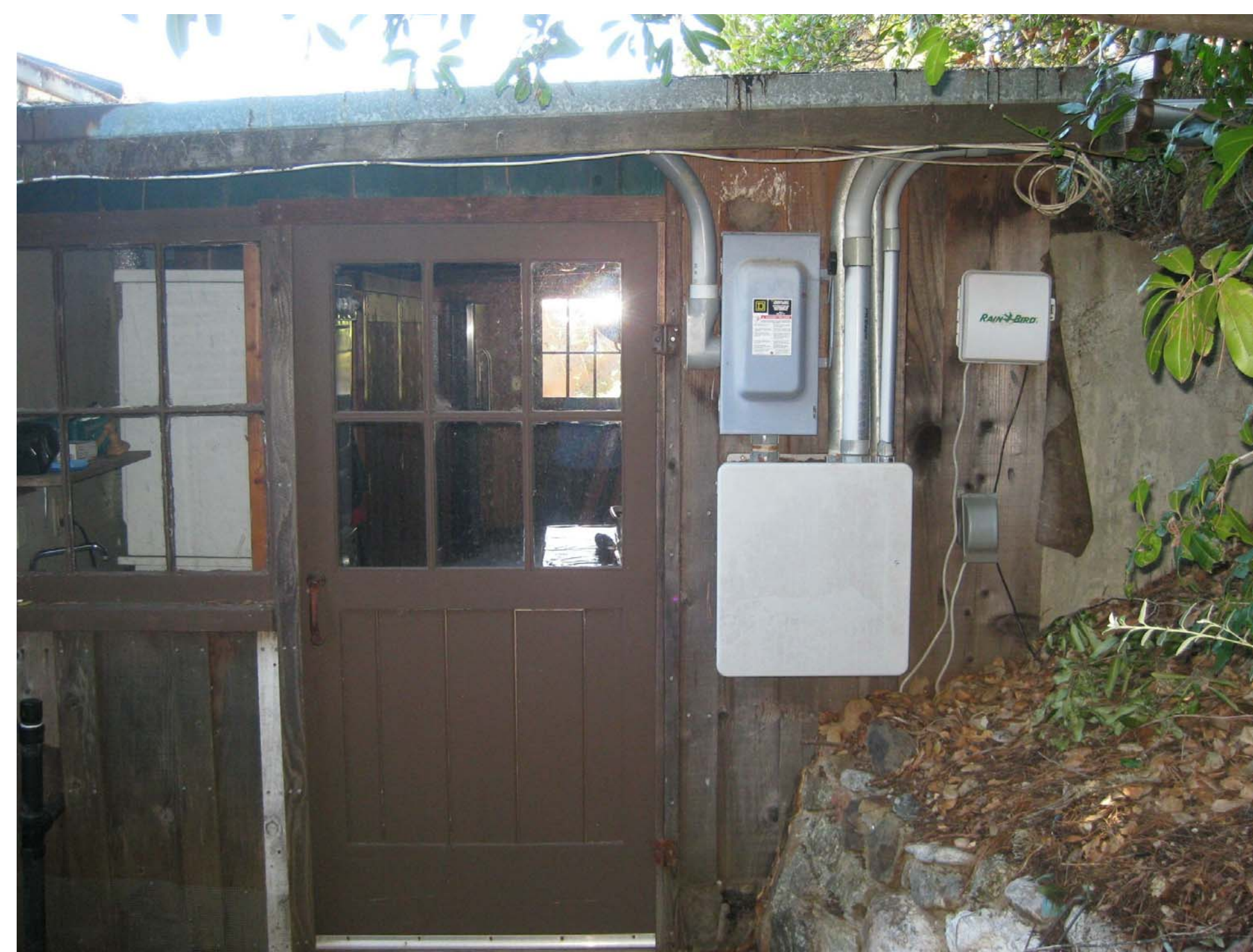
MAIN RESIDENCE - BACK PORCH - N/E ELEVATION
