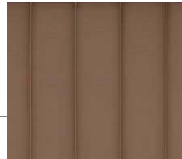
STANDING SEAM COPPER ROOF
