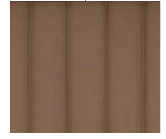
STANDING SEAM COPPER ROOF
