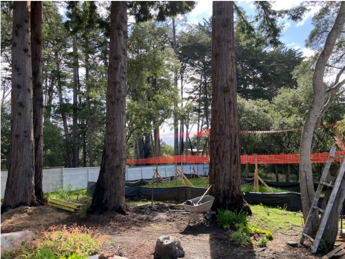
Figure 6. Per the design plans and given the proper installation, maintenance and monitoring of tree protection fencing, the health of the subject redwoods will not be adversely affected by the ADU due to a floated foundation and the trees are not expected to be a hazard concern to nearby structures.
