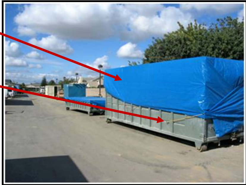
Waste bin with a tarp cover.
