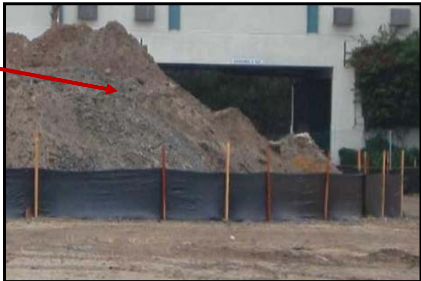
Silt fence as stockpile perimeter control.
