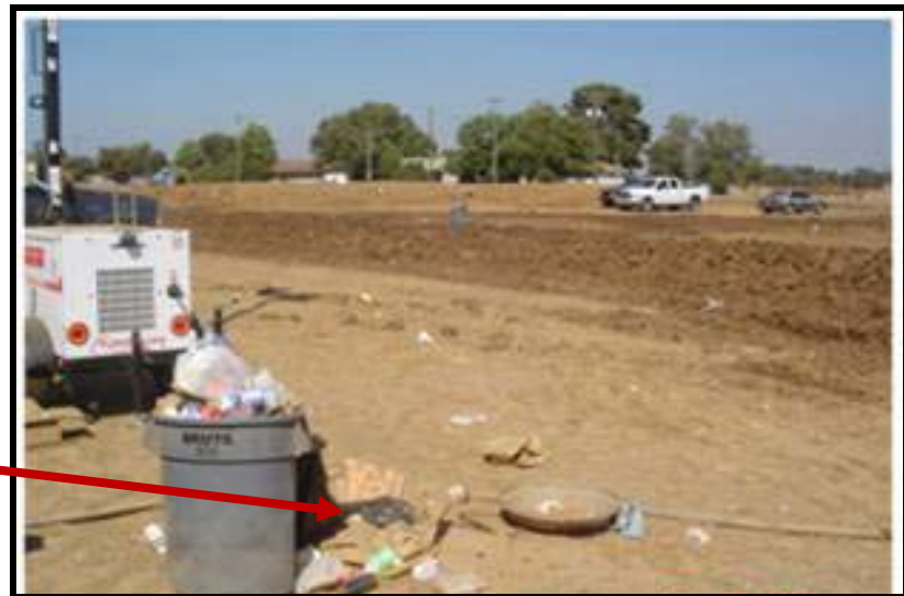
Improperly managed waste receptacle.
