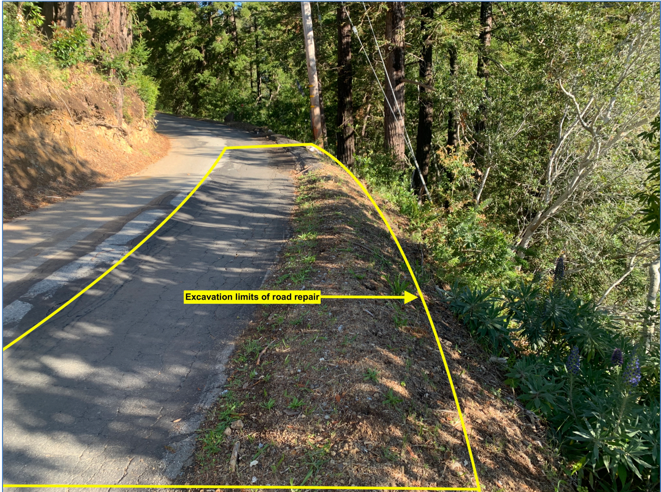
Lower section of proposed hilfiker road repair (April 23, 2026).
