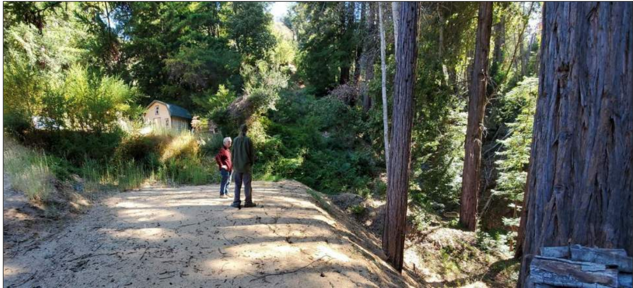
Figure 15 – Fresh veneer of soil on right edge of lower parking pad. Parking area was previously devoid of vegetation, however soil was placed along the right (southerly) side and allowed to cascade down slope. This resulted in covering approximately 400 square feet of Redwood Forest understory with a thin veneer of native soil.
