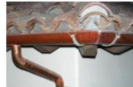
2 COPPER GUTTER & DOWNSPOUT
