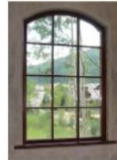
5 WOOD WINDOWS & DOORS
