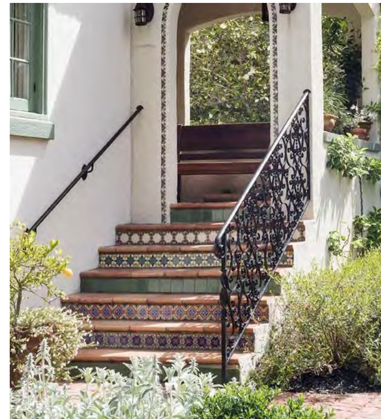
6 EXTERIOR STAIRS & RAILING WHITE W/ WHITE TRIM
