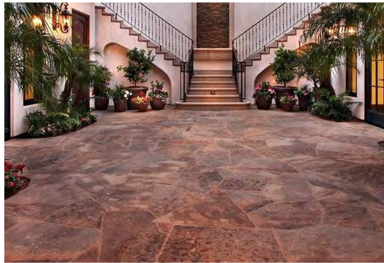
11 PAVING AT FRONT COURTYARD RED SANDSTONE
