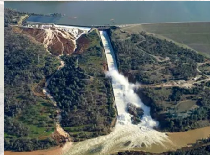
Photos of Oroville Spillway Failure 2017
