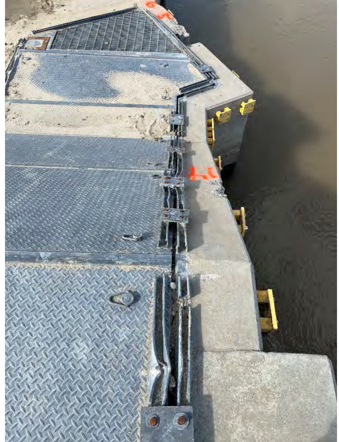
Bent Fish Ladder Top Panels (Three panels damaged)
