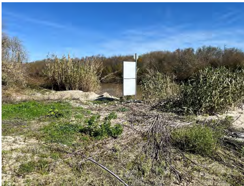
Figure 5: Downstream signage, vegetation removal needed.
