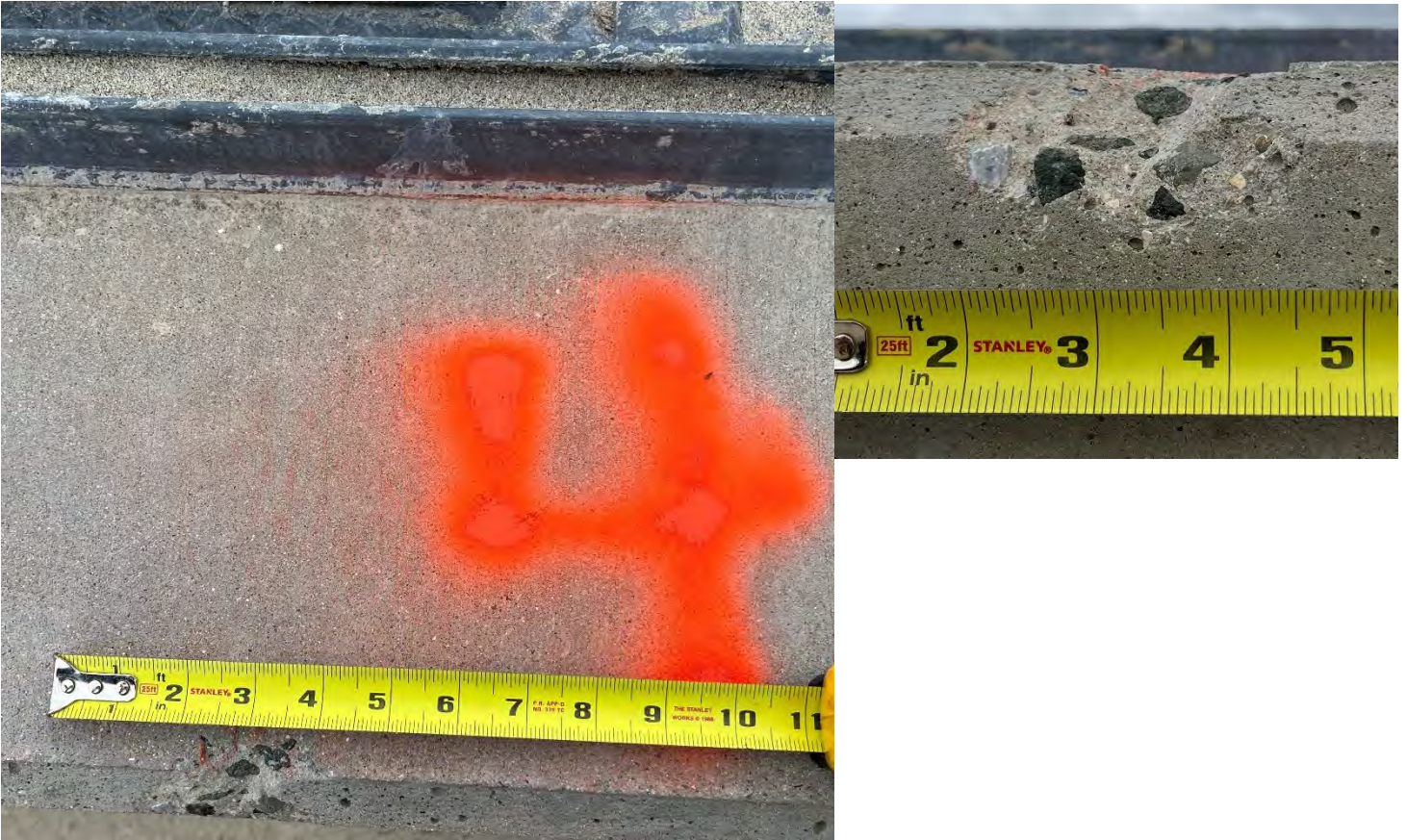
Site #4 Fish Ladder top panels, Left Bank, AOR (9 sq inches)
