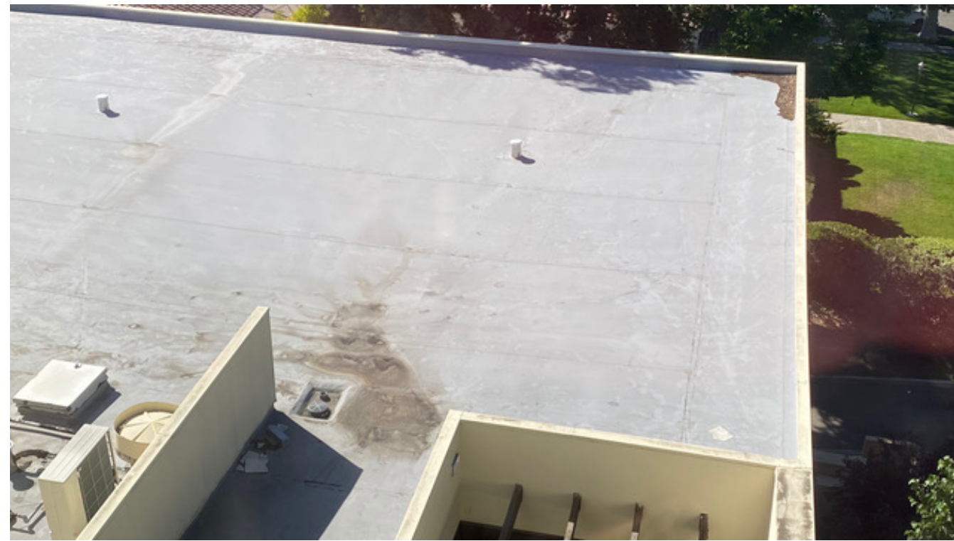
TPO FLAT ROOFING EXAMPLE
