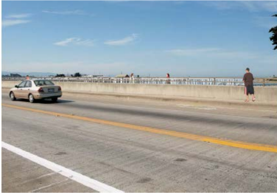
Pedestrians traveling to the southwest towards Moss Landing Harbor and Monterey Bay from the north end of State Highway 1 Bridge crossing Elkhorn Slough
