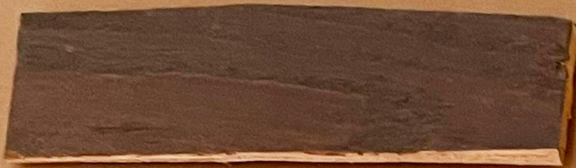
rafter tail & beams
