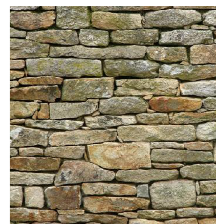
STONE CLAD RETAINING WALL
