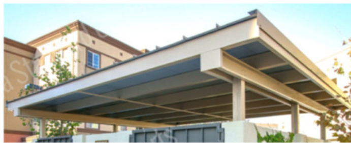
Trash enclosure roof:
