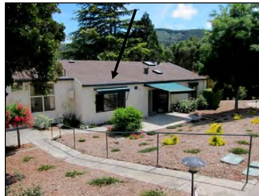
Figure 38. Rear of Bldg. 29 showing garage conversion.
