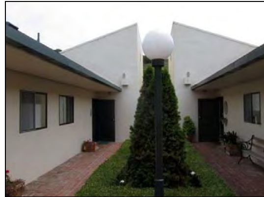
Figure 33. Courtyard of Bldg. 7.
