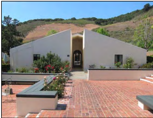
Figure 29. Front (south) elevation of the Bldg. 8.
