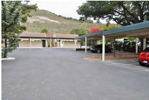
Figure 12. View of upper guest cottages and carport structure to be removed.
