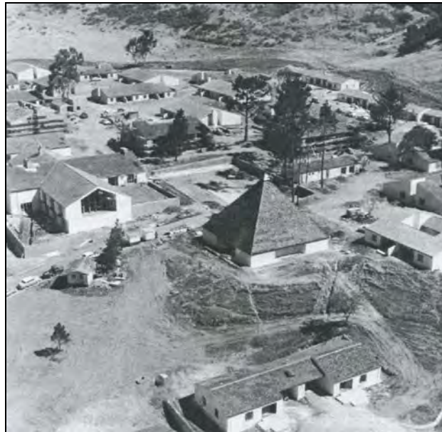
Figure 39. View of Carmel Valley Manor after completion of the buildings. ( Courtesy, Carmel Manor: A History, pp. 21 ).
