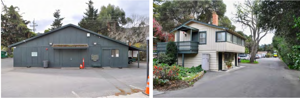
Figures 6 and 7. Left: north elevation of the Wood Shop/Maintenance Shed. Right: south and west elevations of the Lower Guest Cottage.
