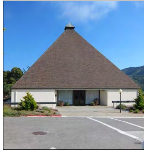
Figure 22. Front (north) elevation of Meeting House.
