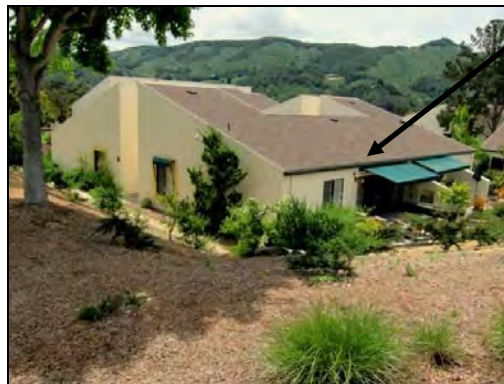
Figure 34. Overall view of Bldg. 18 with full outer wall extension (arrow).
