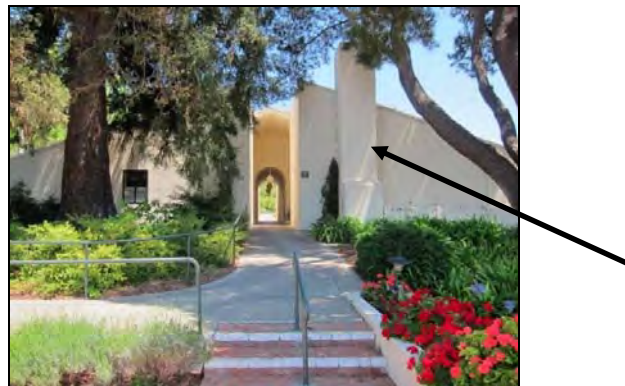
Figure 31. Front (west) elevation of Bldg. 2. Note chimney (arrow) and window in left shed end.
