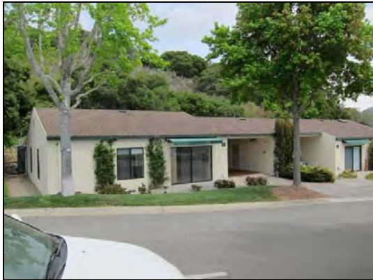
Figure 35. Front (west) elevation of the Bldg. 22.
