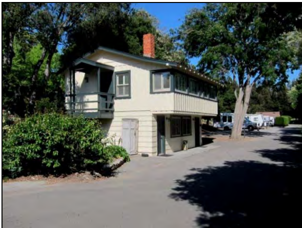
Figure 16. Guest Quarters located off of the service road at the southeast corner of the site.
