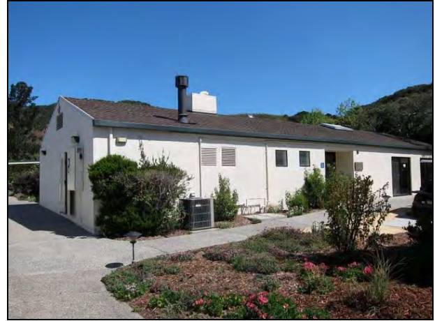
Figure 24. Rear (south) elevation of the Fitness Center.
