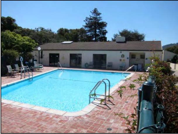
Figure 23. Front (north) elevation of the Fitness Center.
