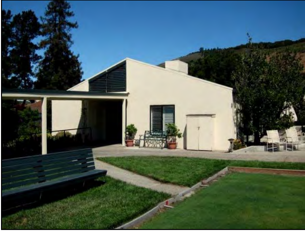
Figure 25. Front (south) elevation of the West Parlor. Note the covered walk leading to the façade.
