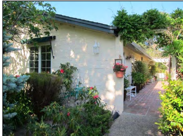
Figure 15. Bldg. 25 constructed of adobe.
