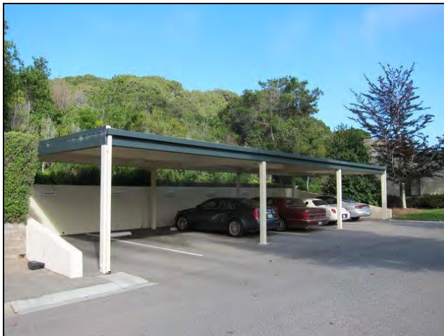
Figure 12. Typical covered parking area.
