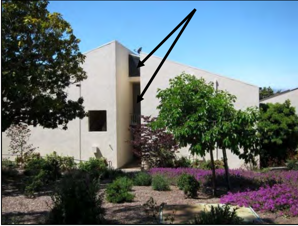
Figure 27. Rear (east) elevation of the Bldg. 17. Louvered vent and glazing alteration shown with arrows.
