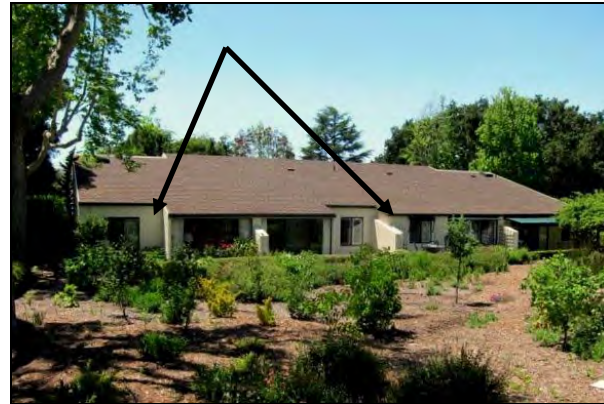
Figure 30. Bldg. 3 outer wall extensions shown with arrows.
