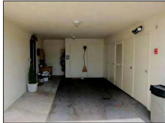
Figure 36. Typical garage design seen on Bldg. 22.
