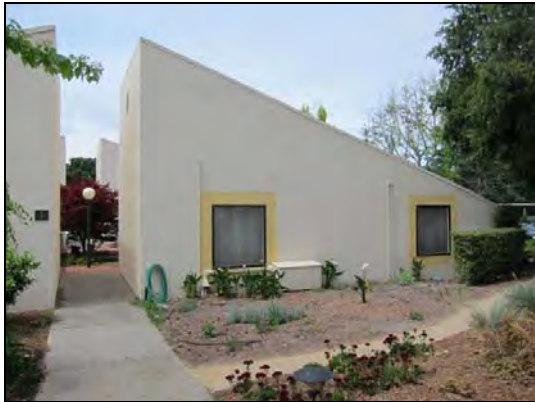
Figure 32. Front (east) elevation of the Bldg. 4.
