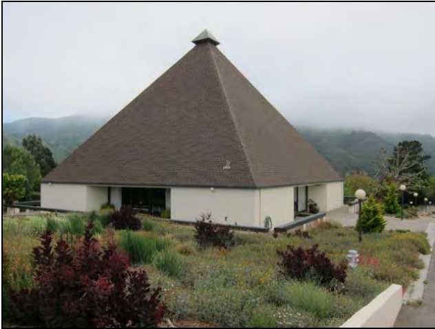
Figure 21. Side (east) elevation of Meeting House.
