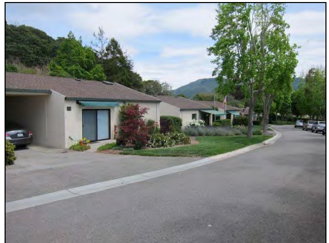
Figure 9. Arrangement of duplex units along upper Carmel Valley Manor Road.
