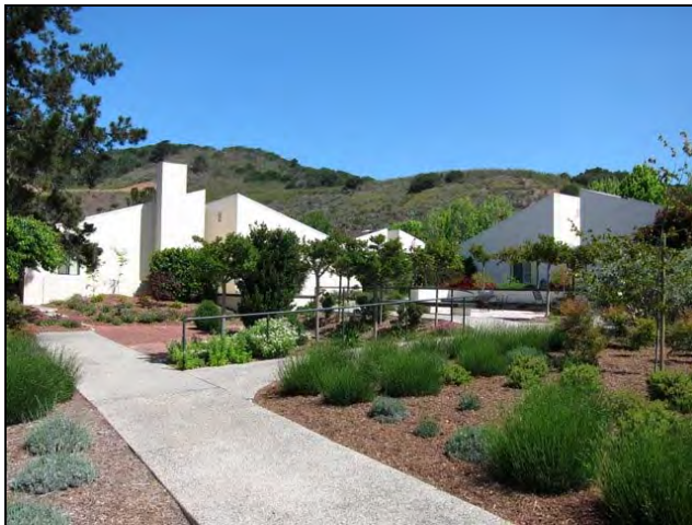
Figure 8. Typical cluster of buildings around open courtyard.
