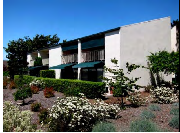
Figure 28. Side (north) elevation of Bldg. 14.
