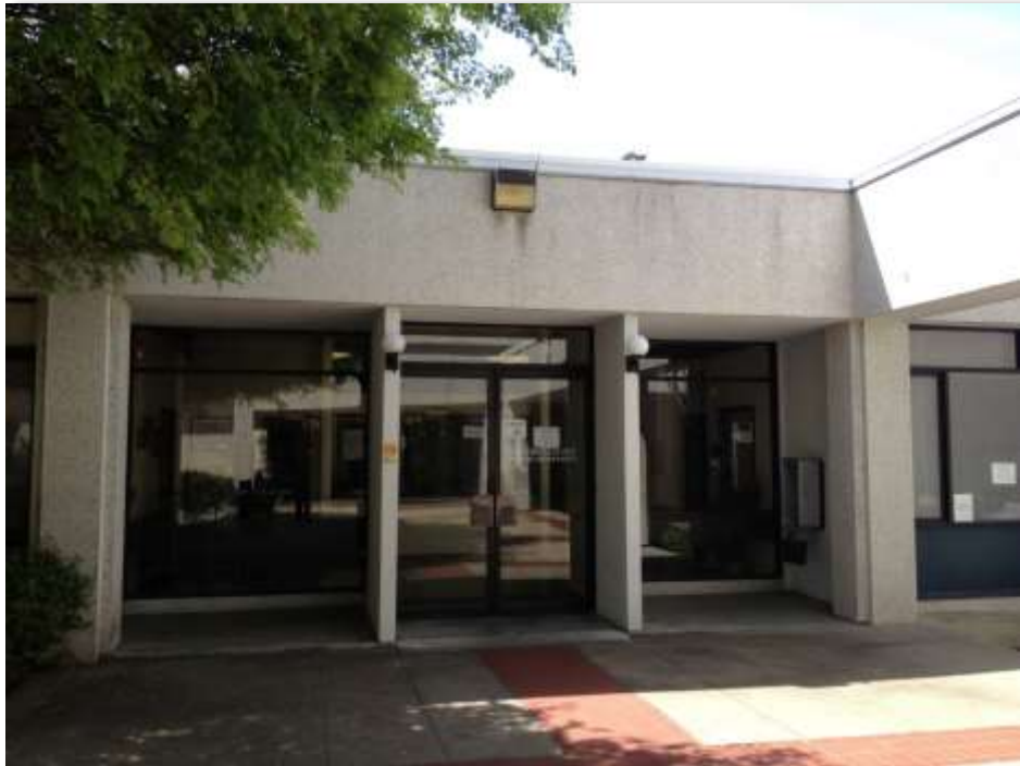
Exterior- Entry to Monterey County Health Services Department
