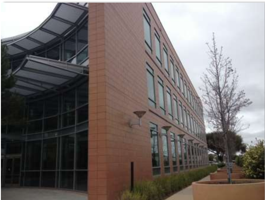
Exterior – East Side
