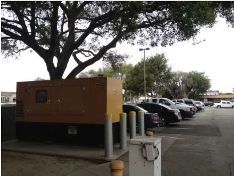
Exterior – Rear Parking Area
