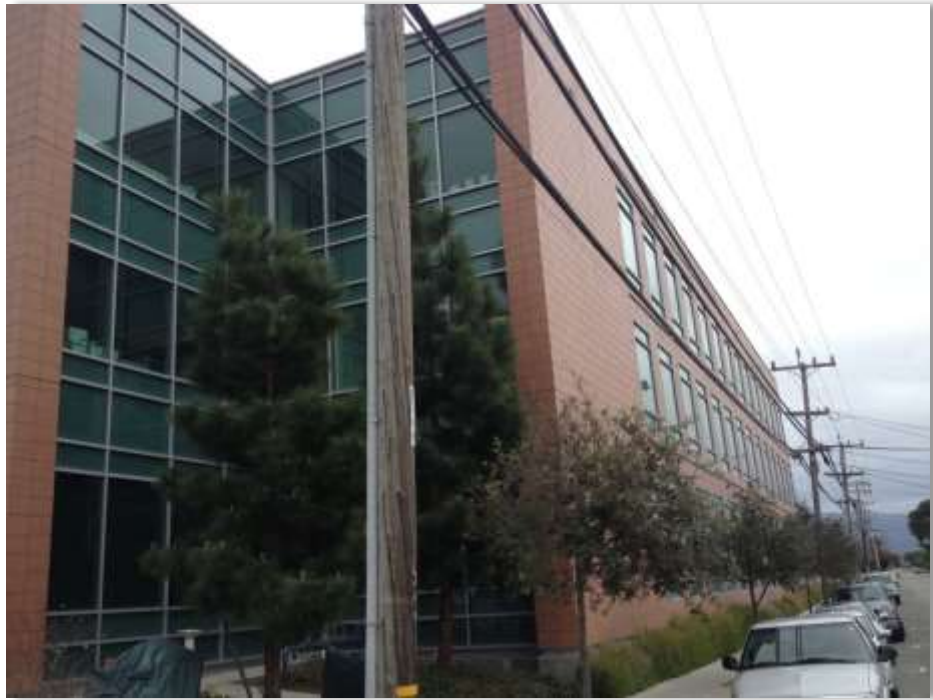
Exterior – West Side
