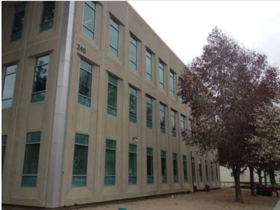
East Side of Courthouse
