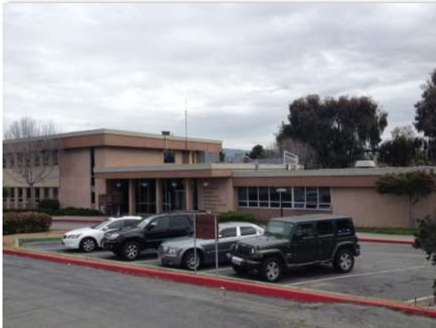
Front Exterior - Entry
