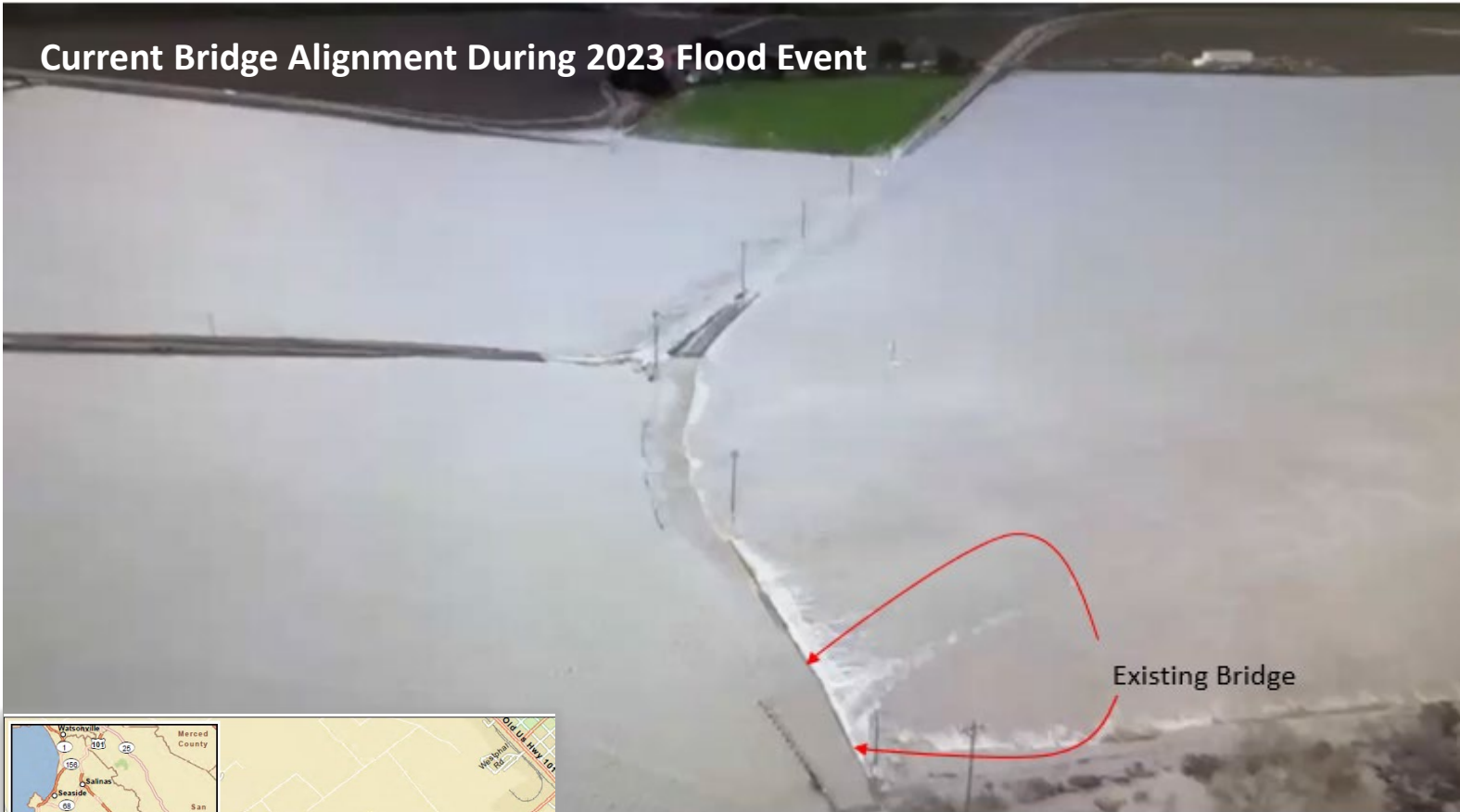
Flood Waters Undermined Bridge in 2023
