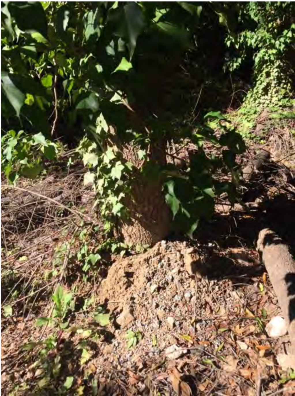
Figure 11. One of a few examples where fill material is smothering the lower trunk and root crown of roadside trees.
