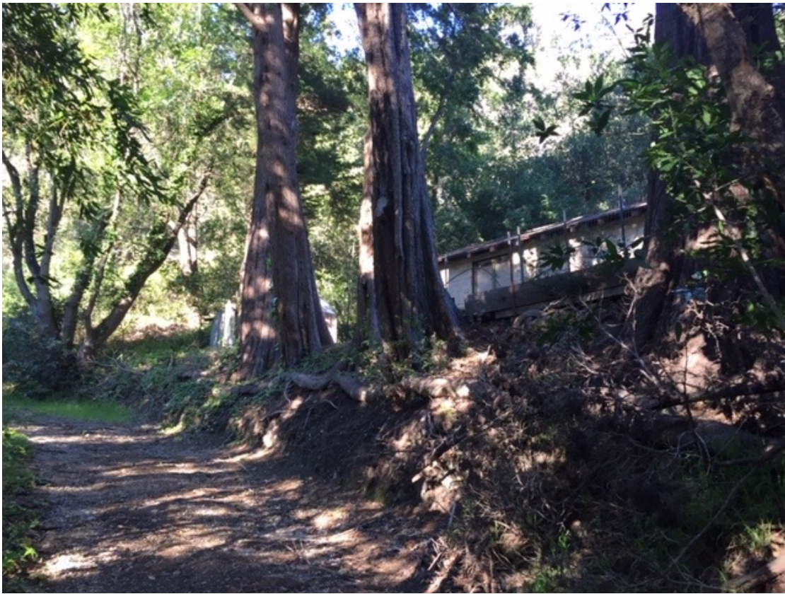
Figure 9. Blaze Engineering apparently cut in this non-permitted road just below the Donaldson's cabin, which resulted in several large roots being cut and damaged on the upper cut slope. This area is located just above the proposed office building.
