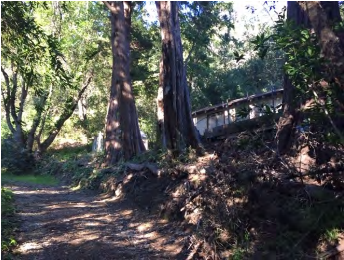
Figure 9. Blaze Engineering apparently cut in this non-permitted road just below the Donaldson's cabin, which resulted in several large roots being cut and damaged on the upper cut slope. This area is located just above the proposed office building.
