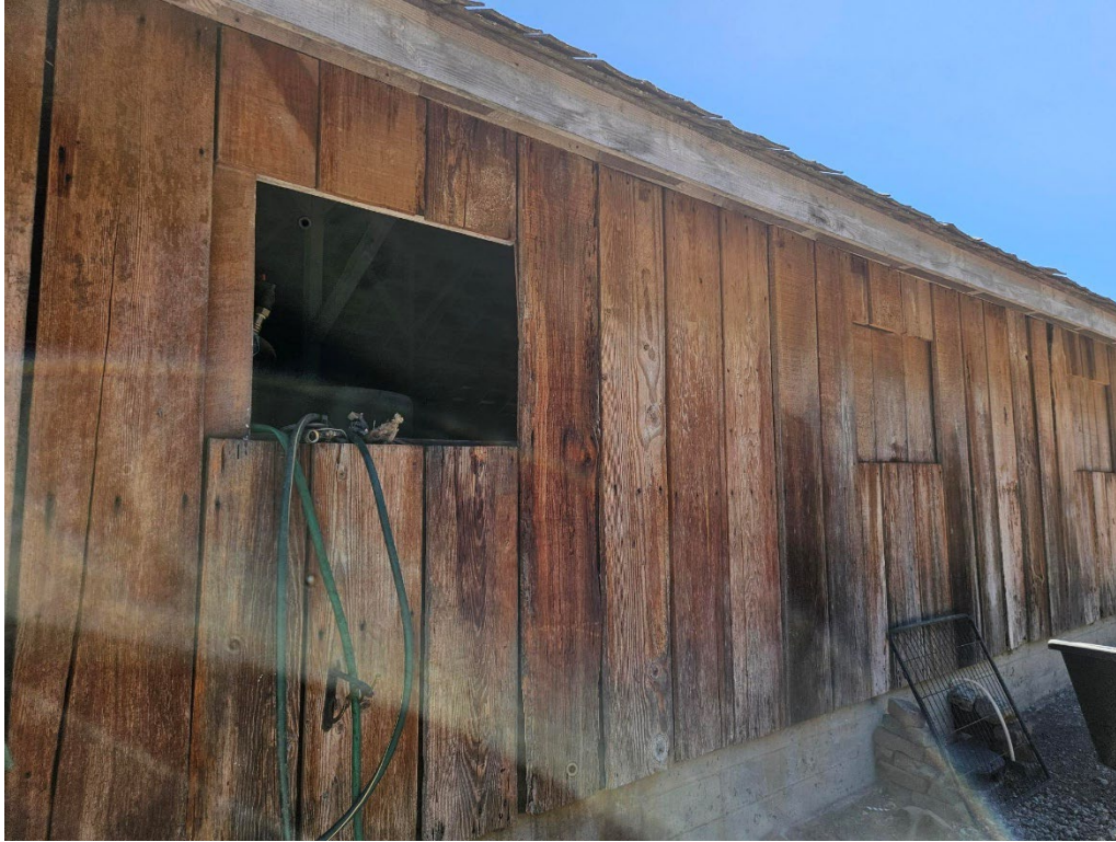
Figure 5: Detail of stall windows, opened and closed with sliding wood shutters.
