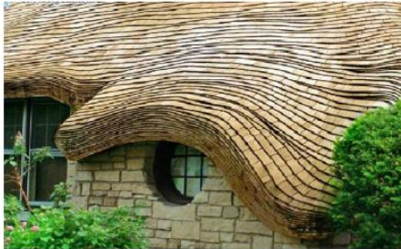
Steamed rolled cedar shingle roof with natural finish
