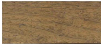
Stained wood soffits, garage doors, trims
