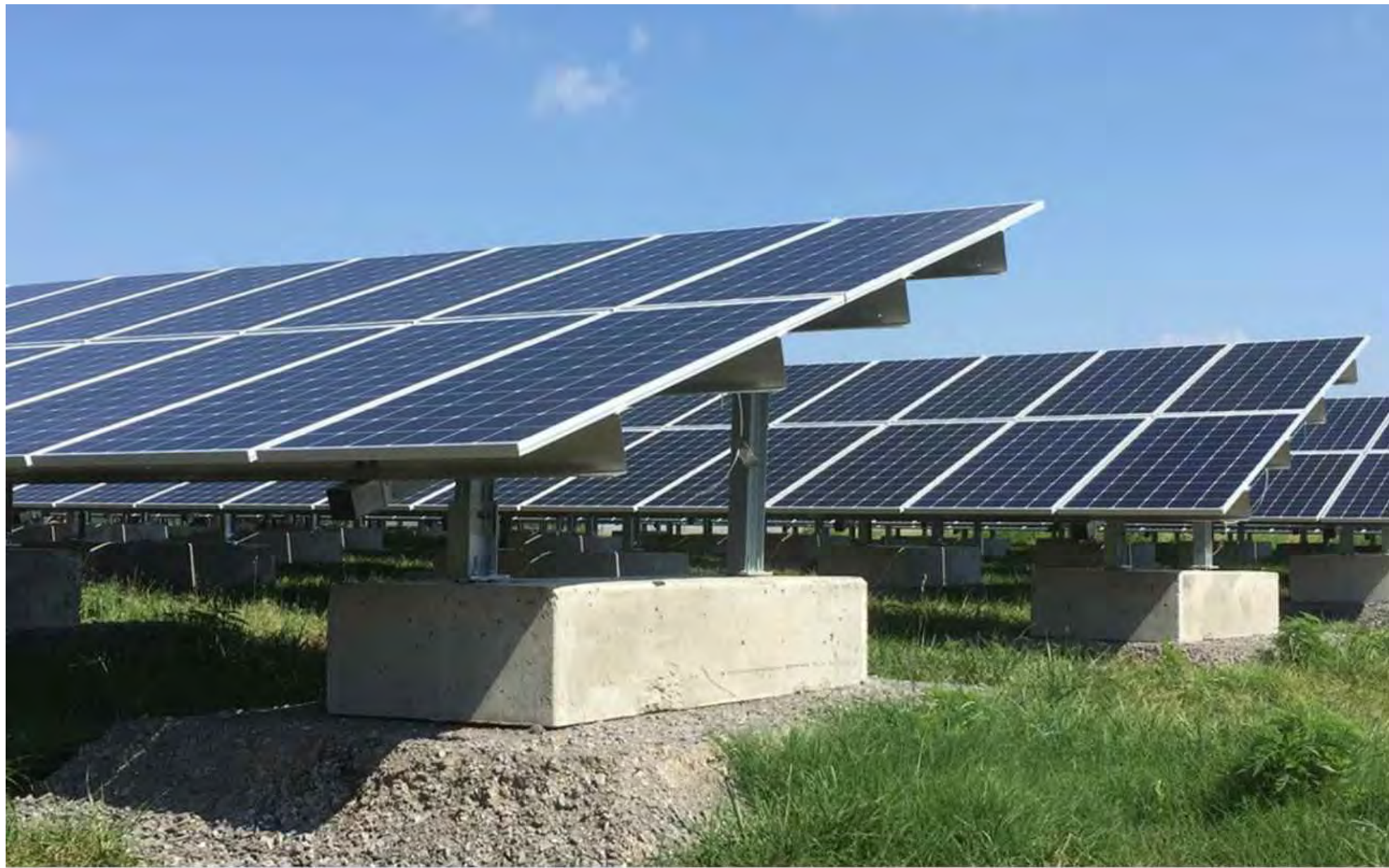
TYPICAL FIXED TILT RACKING ON BALLASTED FOUNDATIONS
