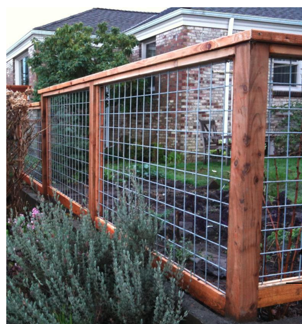
NEW FENCE CONCEPT NEW FENCING AT SIDE AND REAR PROPERTY LINES. WOOD & WIRE DEER FENCING 6'-0" MAX. HT.
