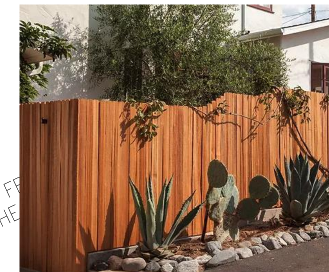
NEW FENCE CONCEPT NEW FENCING AT FRONT PROPERTY LINE. MODERN GRAPE STAKE 4'-0" MAX. HT.
