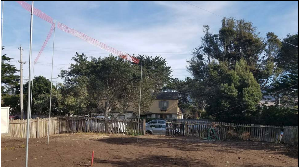
Figure 14a – Site Visit Photos: Staking and Flagging at 26338 Valley View Avenue
