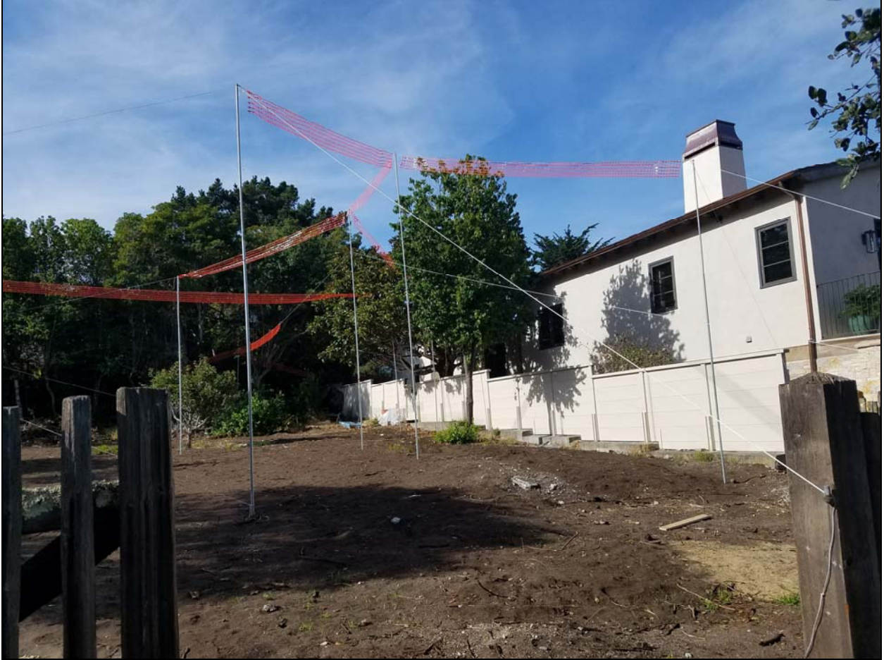
Figure 15a – Site Visit Photos: Staking and Flagging at 26338 Valley View Avenue
