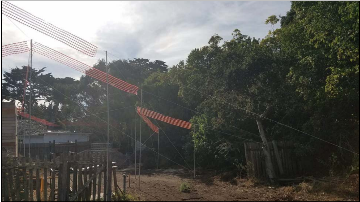
Figure 14b – Site Visit Photos: Staking and Flagging at 26346 Valley View Avenue
