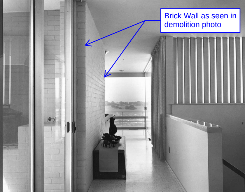
View from landing looking South
