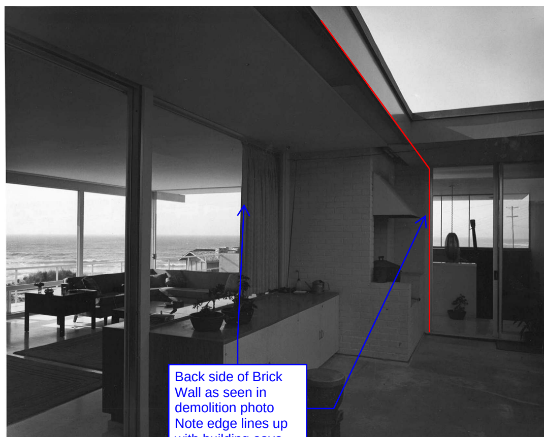
View from Courtyard looking West
