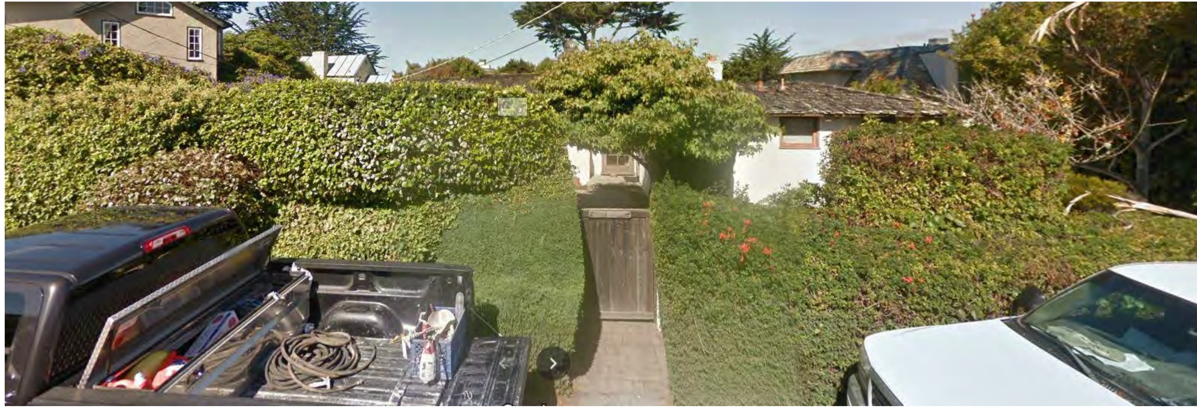
1 SOUTH ELEVATION - ENTRY TO SITE
