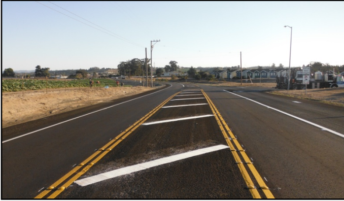
Castroville Blvd. Overlay/Pavement Delineation
