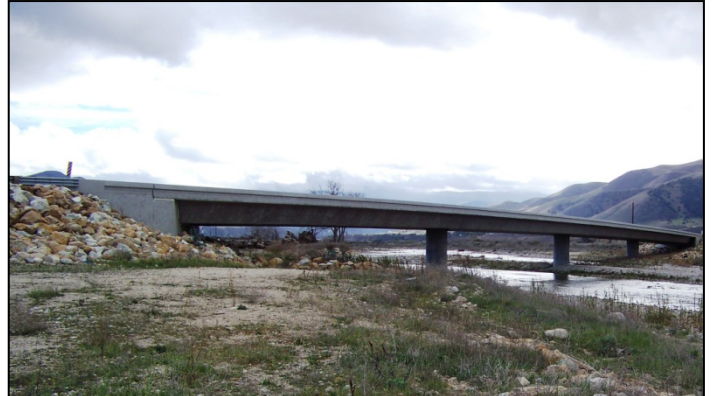
Thorne Road Bridge
