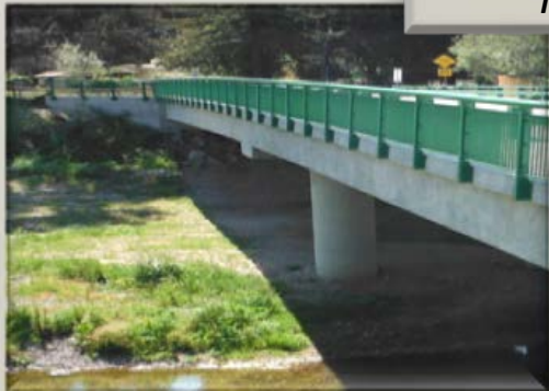
Schulte Road Bridge
