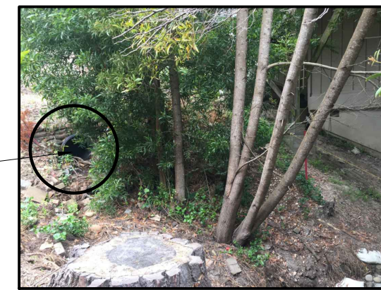
EXISTING MONTEREY COUNTY MAINTAINED STORM WATER DRAINAGE 24" CULVERT OUTLET CAUSING SEVERE EROSION AND DAMAGE TO BUILDING FOUNDATIONS OF THE KOSTIGEN RESIDENCE
