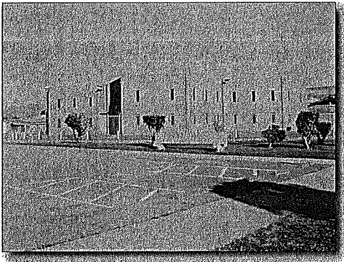
The Monterey County Main Jail.
