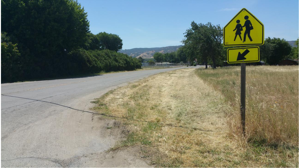
Center St./Cattlemen Rd. intersection looking West (San Ardo)
