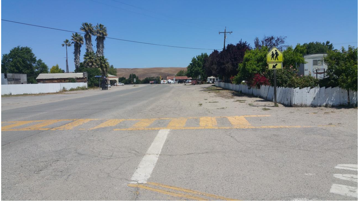
Center St./Cattlemen Rd. intersection looking East (San Ardo)
