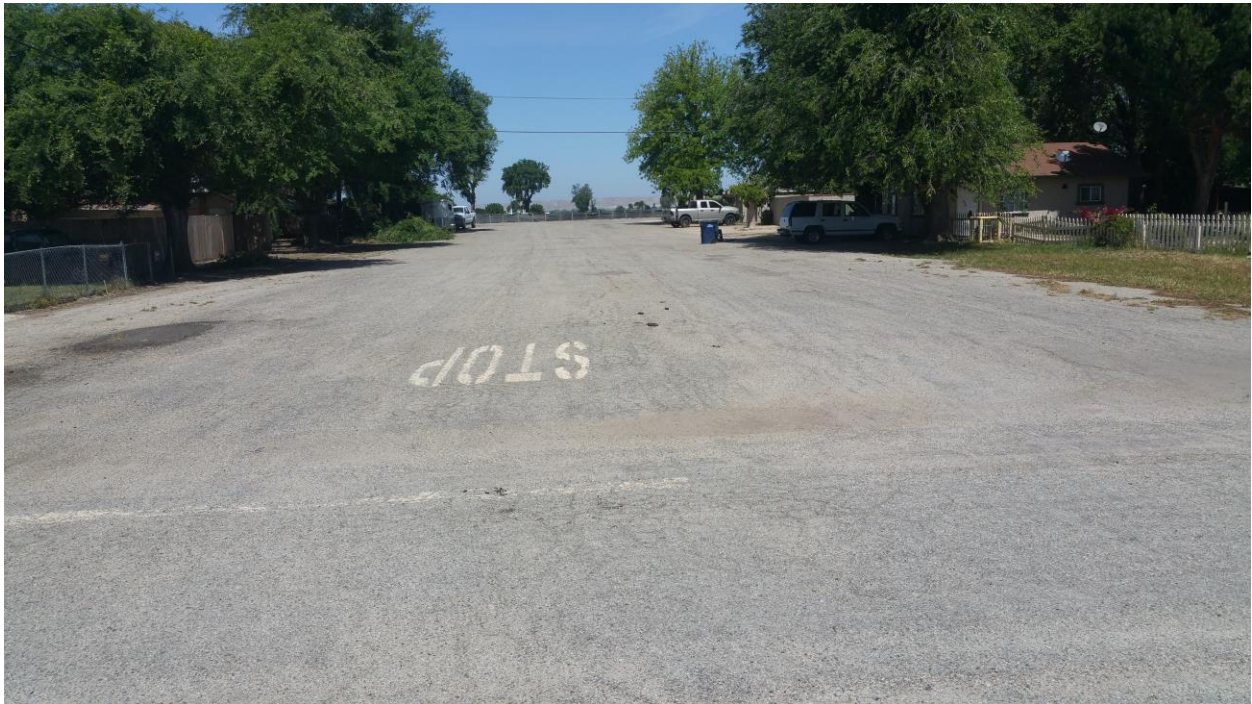
College St./Martin St. intersection looking North (San Ardo)
