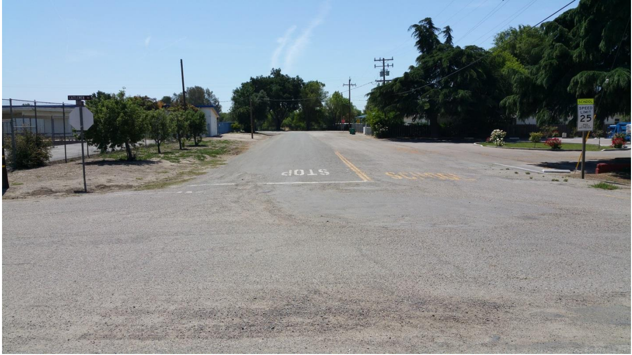
Godchaux St./College St. intersection looking South (San Ardo)
