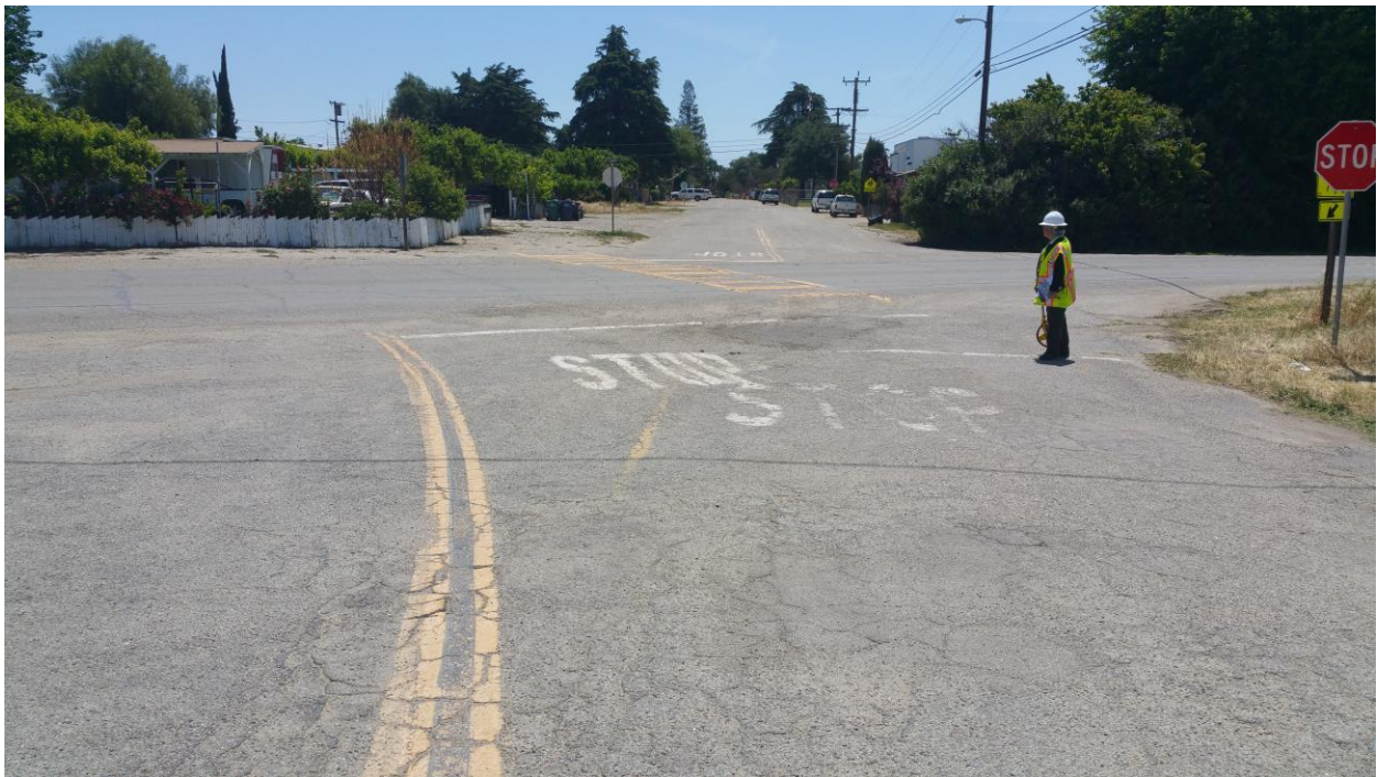
Center St./Cattlemen Rd. intersection looking South (San Ardo)
