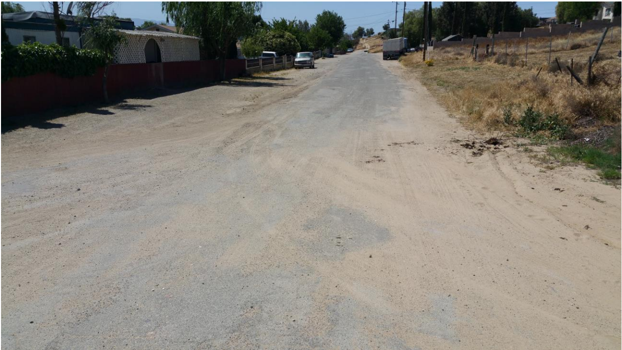
Anita St./San Benito St. intersection looking West (San Lucas)
