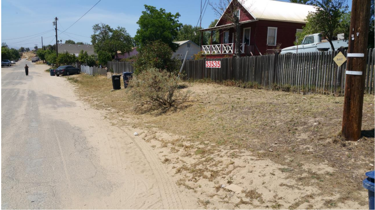
Teresa St./San Benito St. intersection looking West (San Lucas)
