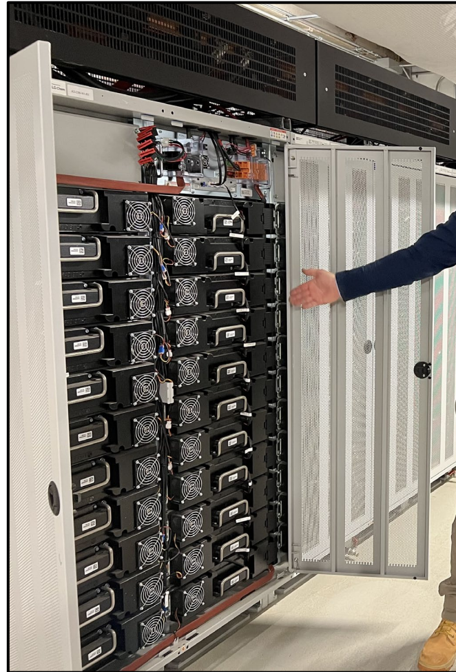
Battery Rack (22 Modules)
