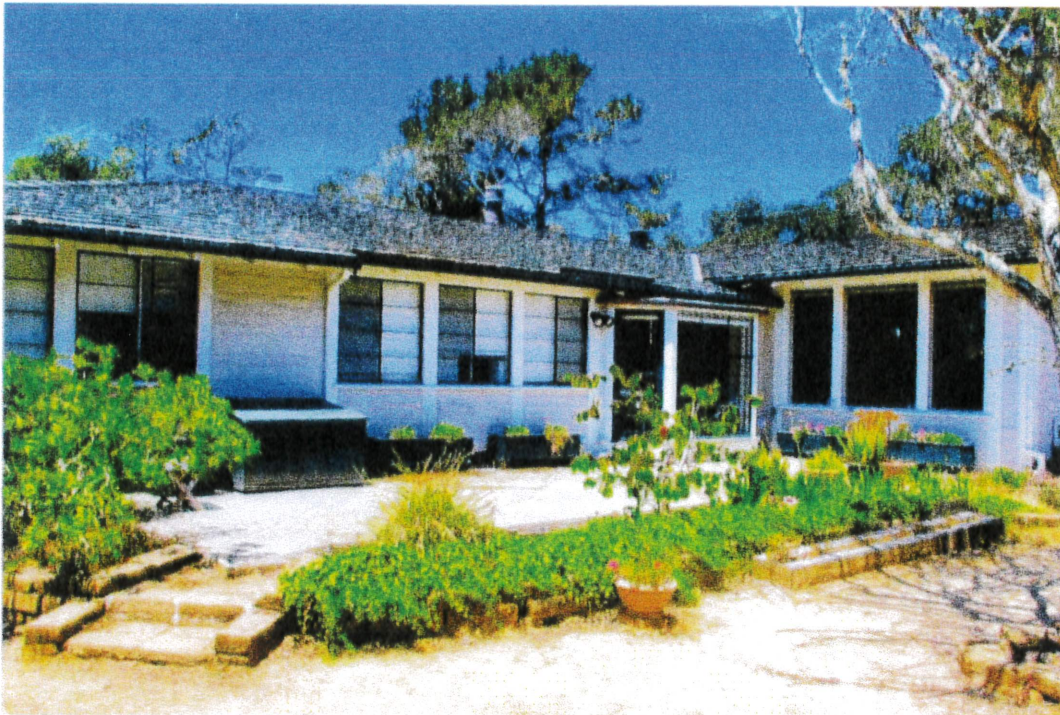
Photo #4. Looking NE at the South side elevation, note angled c. 2007 bay to right & c. 2003 in filled chimney at left, Kent Seavey, Dec., 2022.
