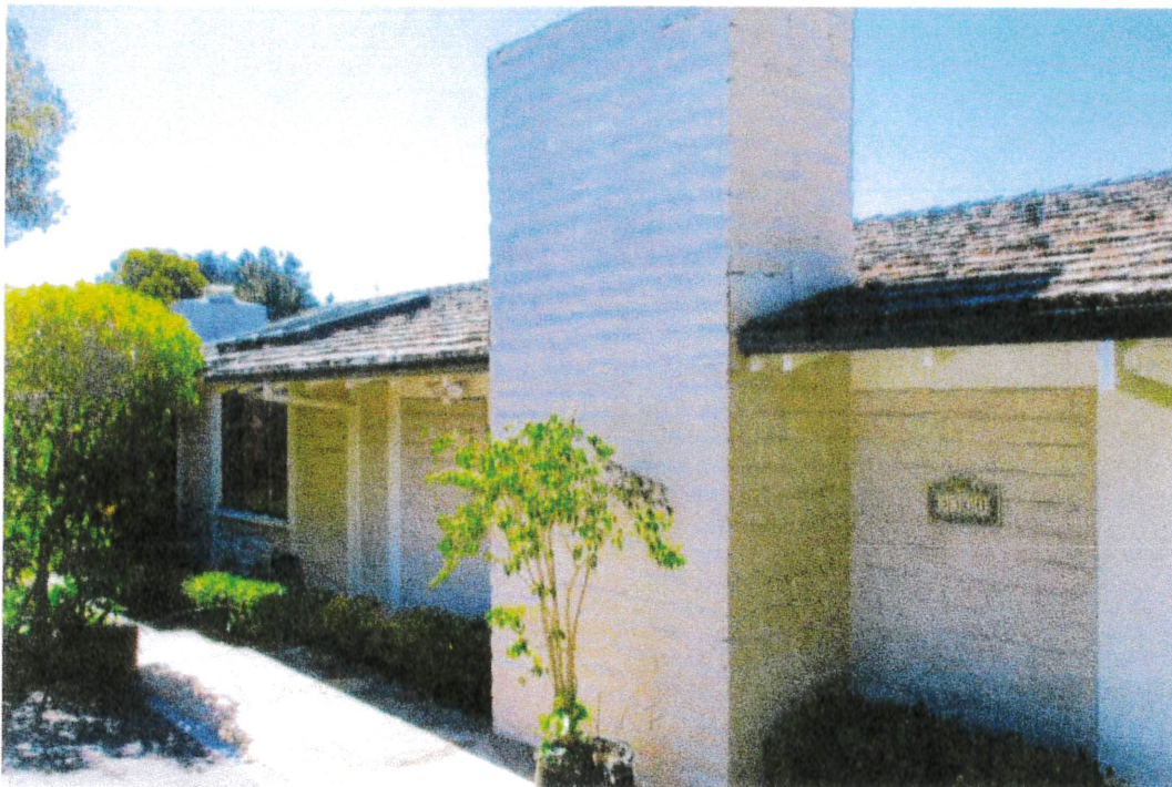
Photo #2, Looking SE at North facing facade, note c.1953 in fill of original garage for bedroom space, Kent Seavey, December, 2022.
