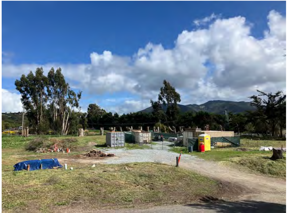
Figure 24. This impacted and disturbed area at the lower southeast end of the CVM property will be a parking area. No native species trees that have County protection status will be impacted or removed.
