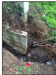
EXISTING MONTEREY COUNTY MAINTAINED STORM WATER DRAINAGE CHANNEL CAUSING SEVERE EROSION AND DAMAGE TO BUILDING FOUNDATIONS.
