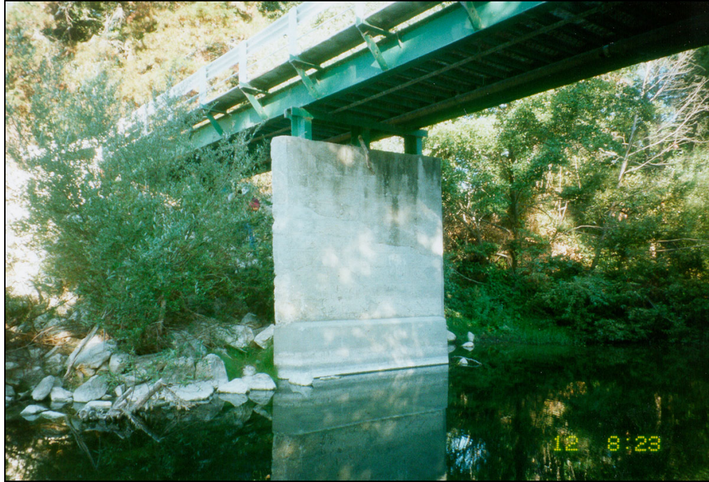
VIEW OF CONCRETE PIER LOOKING SOUTH
