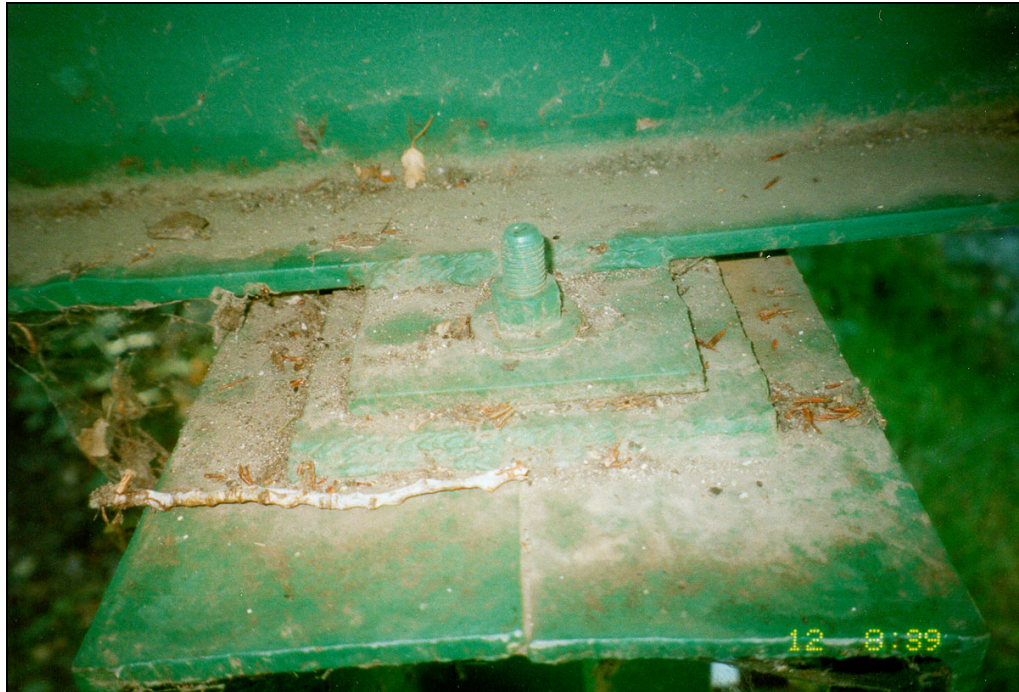
VIEW OF ANCHOR BOLTS UNDER GIRDER
