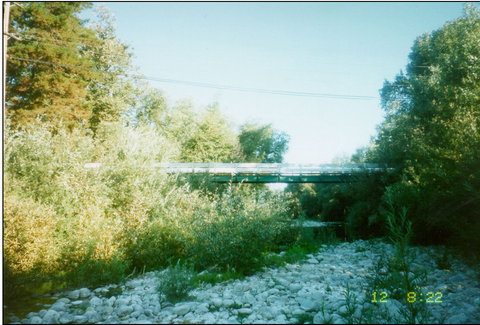
Boronda Road Bridge over Carmel River Br. No. 507 (44C-99)
