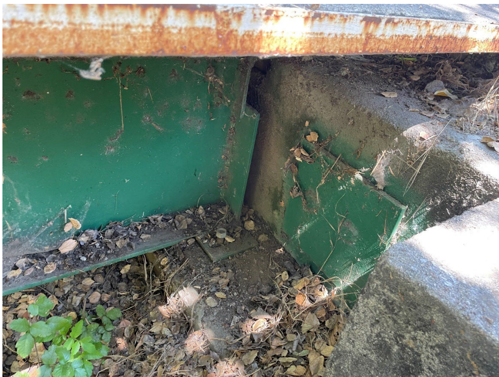
Photo 10: Anchor bolts at east abutment
