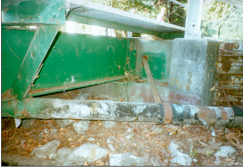
VIEW OF UTILITY PIPE AT SOUTH ABUTMENT
