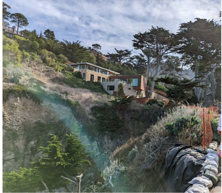
C2) 255 Highway 1 Carmel, CA - Cliff washing out across driveway
