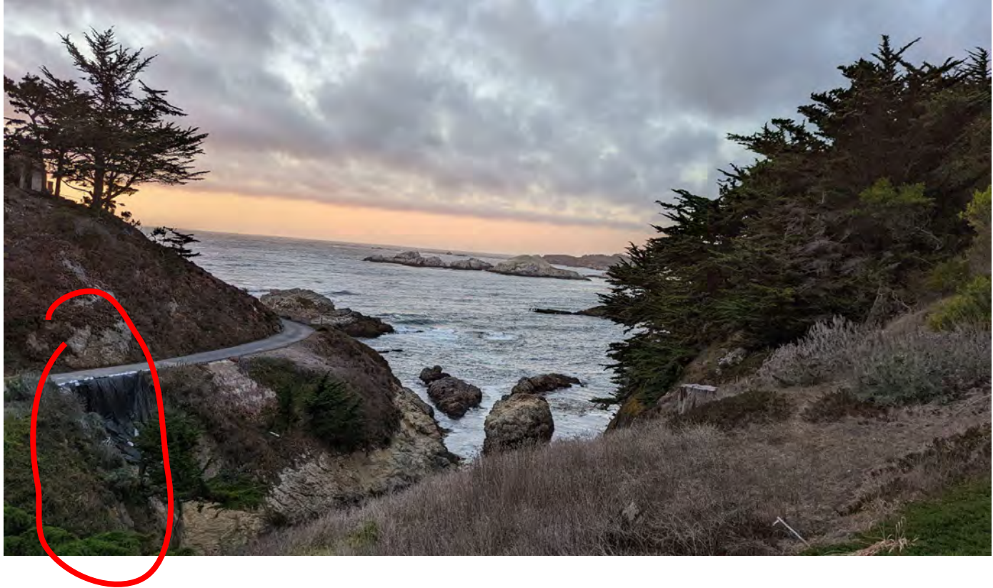
C5) 255 Highway 1 Carmel, CA - Cliff washing out across driveway
