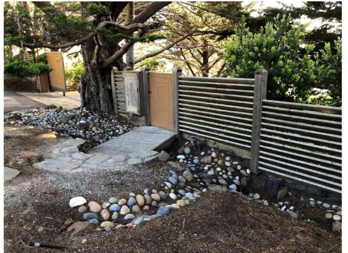
ACCESS DOOR AT MAIN ENTRY GATE
