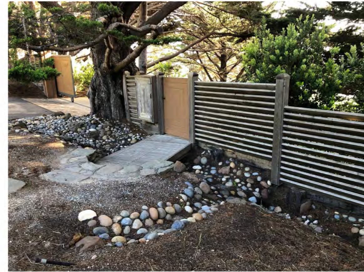
ACCESS DOOR AT MAIN ENTRY GATE
