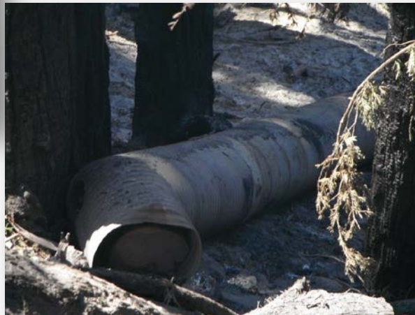
Damaged Culvert
