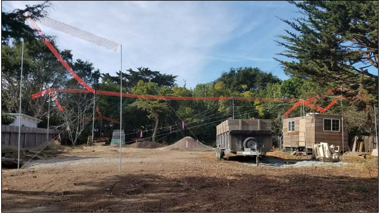
Figure 12b – Site Visit Photos: Staking and Flagging at 26346 Valley View Avenue
