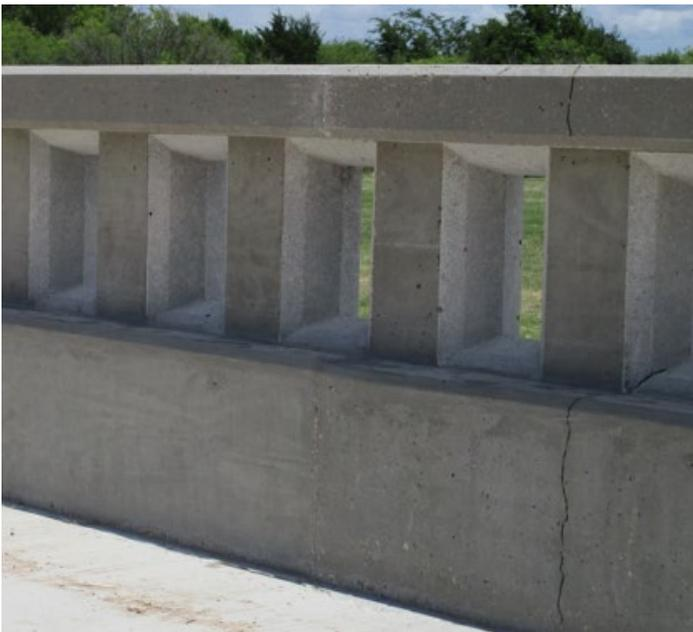
**Figure 2: Texas Department of Transportation Railing with an example photo from outward face of the rail.**
