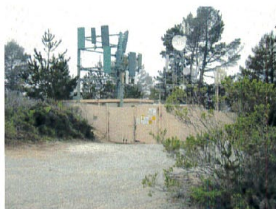
⑤ Cellular communication tower located in north central portion of site near Monterey pine trees
