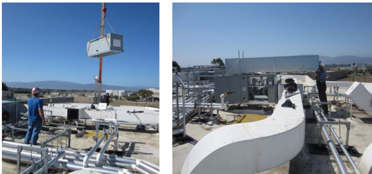
Photo 3-1. HVAC System Retrofits Being Installed at the County Jail
