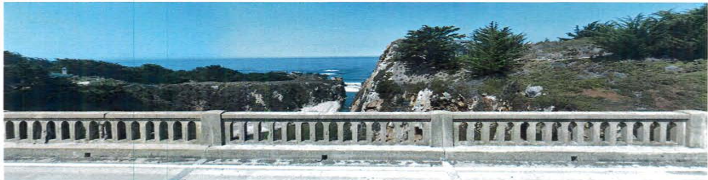
EXISTING ON DECK VIEW
