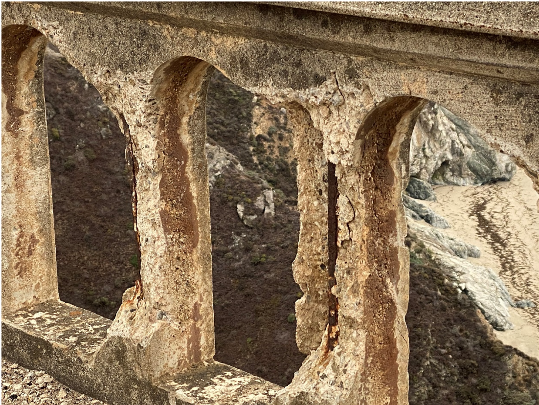
Figure 1-2 Photo of Bixby Creek Bridge Rail Deterioration
