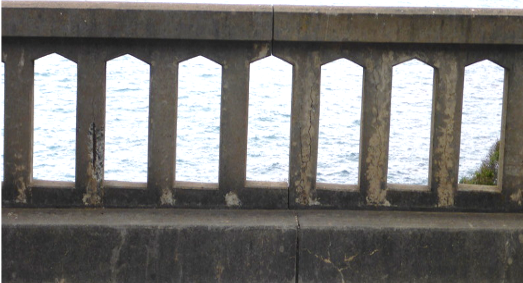
Figure 1-2 Photo of Bixby Creek Bridge Rail Deterioration
