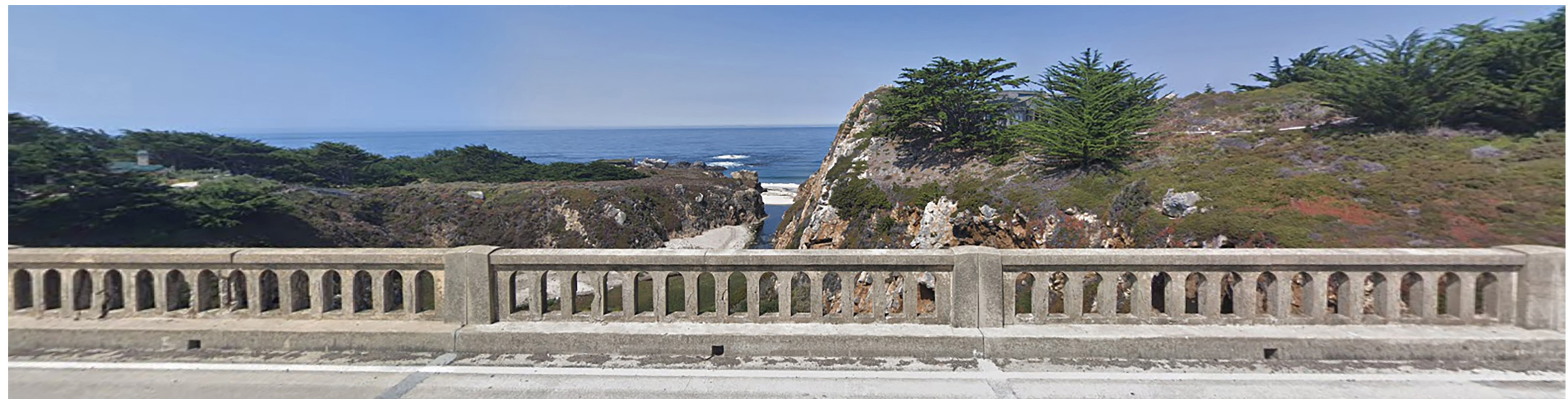
EXISTING ON DECK VIEW
