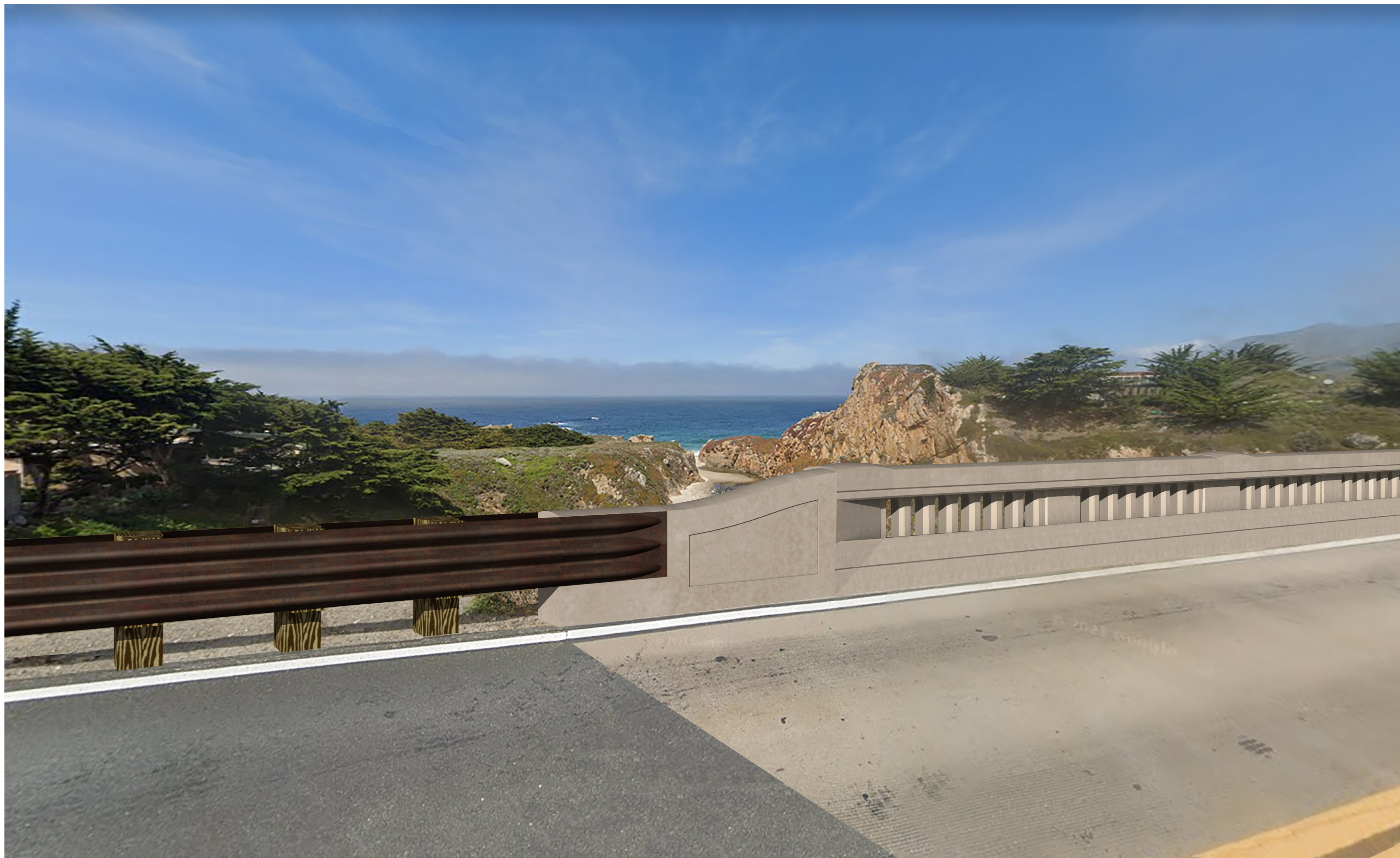
86H SOUTH END BLOCK PHOTO SIM.
